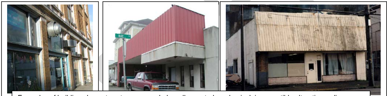
Examples of building elements not recommended: wall mounted mechanical, incompatible alterations, slip cover
